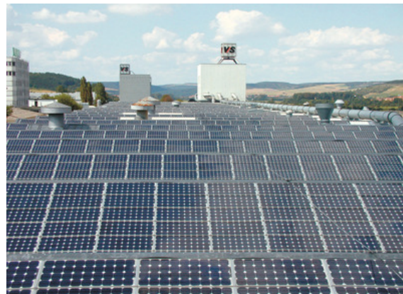
View on rooftops of VS Factory I
